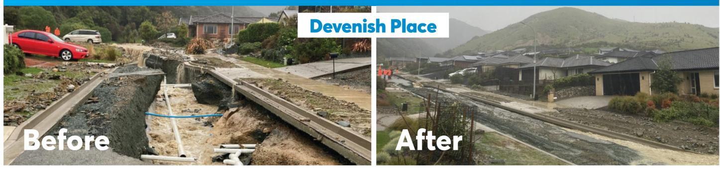
The small, white pipes you can see in the first photograph are for wastewater (the concrete stormwater pipe runs down the road to the left and is much bigger).
