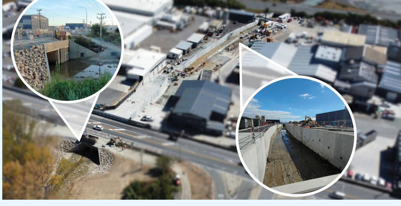
Stage 4 under Main Road Stoke through State Highway 6.
